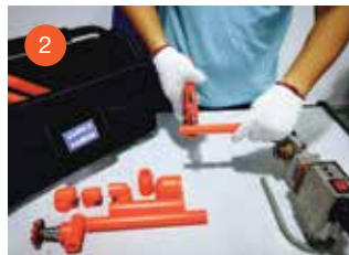
2 Square and prepare the pipe ends.
