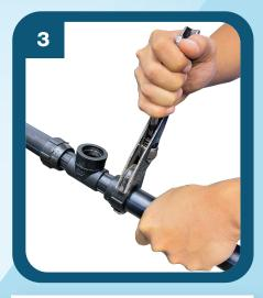
**Step 3**Wind the nut onto pipe a few turns. Tighten it using pipe wrench.
