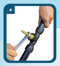
**Step 4**Install cartridge and tighten it using adjustable or ring spanner.
